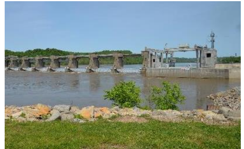
Willow Island Hydroelectric Plant
