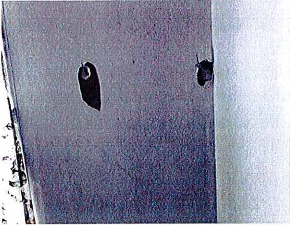
245-2 Bedroom 1 Drywall None Detected
