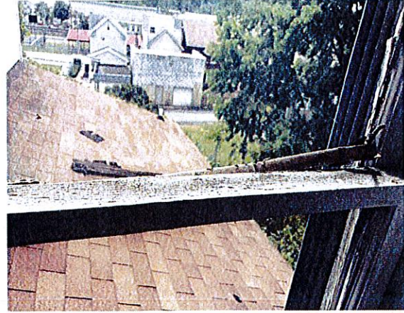
245-3 and 4 Bedroom 2 Interior Window Glazing 18-20%
