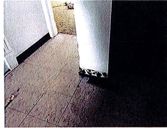
245-6 Kitchen Cove Base and Mastic None Detected
