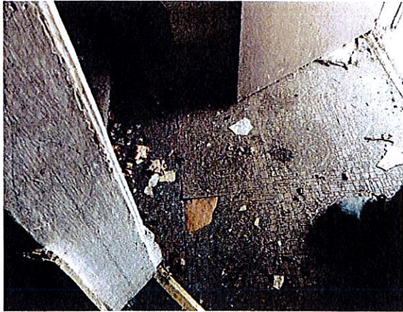
243-7 Entry Floor Tile and Mastic 4-5% in Tile None Detected in Mastic
