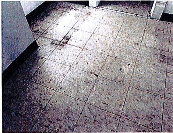
245-5 Kitchen Floor Tile/Mastic/Vapor Barrier 6-7% in White Tile - 7-8% in Grey Tile None Detected in Mastic or Vapor Barrier
