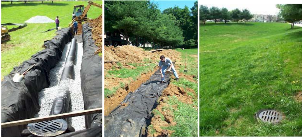
Figure 3: Example of Infiltration Trench Installation
